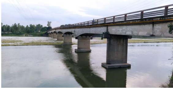
(c) Vushirbandar Bridge: Beam and arch shaped concrete bridge
