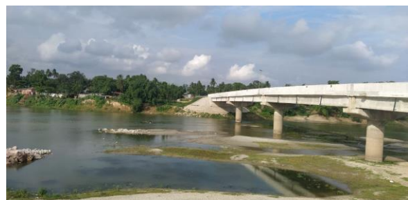
(b) Kakra Bridge: Concrete beam bridge
