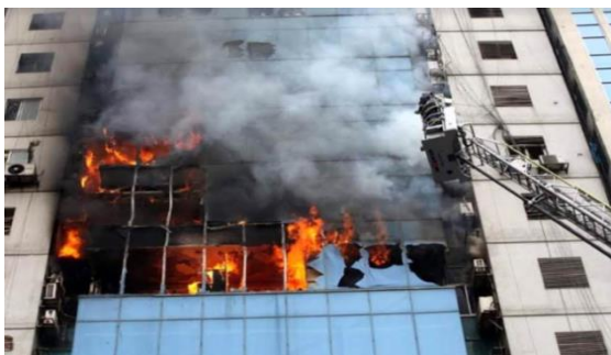
e) Fire on 22 storied F R Tower, Banani, Dhaka (on March 28, 2019)
