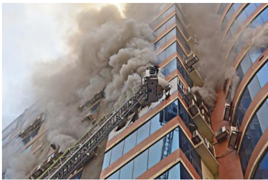
c) Fire on 15 storied Zaman Tower, Paltan, Dhaka (on Dec 29, 2018)
