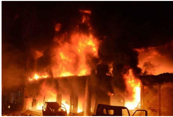
a) Fire at Nimtoli, Dhaka (June 2010)
