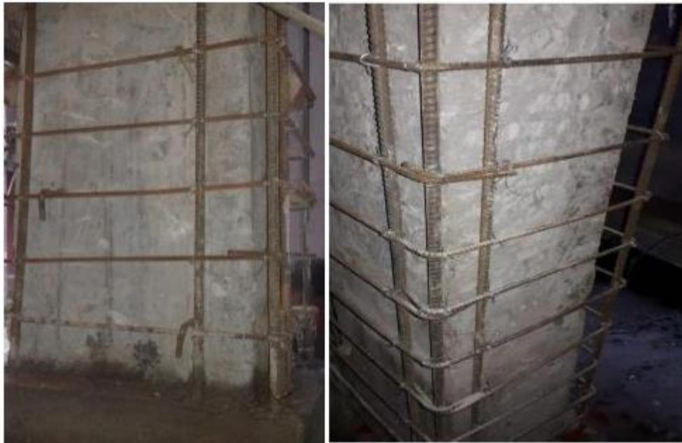
Figure 15: Photos of RCC column jacketing construction.
