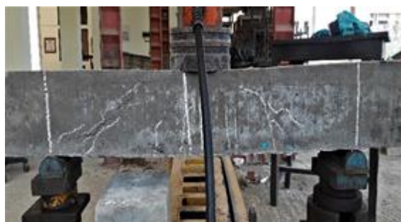
(c) Cracks in 2% polypropylene fiber beam
