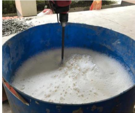
Figure 1: Mixing procedure of foamed concrete
