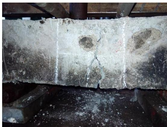
Figure 5: Spalling of concrete in the beam due to burning in fire.
