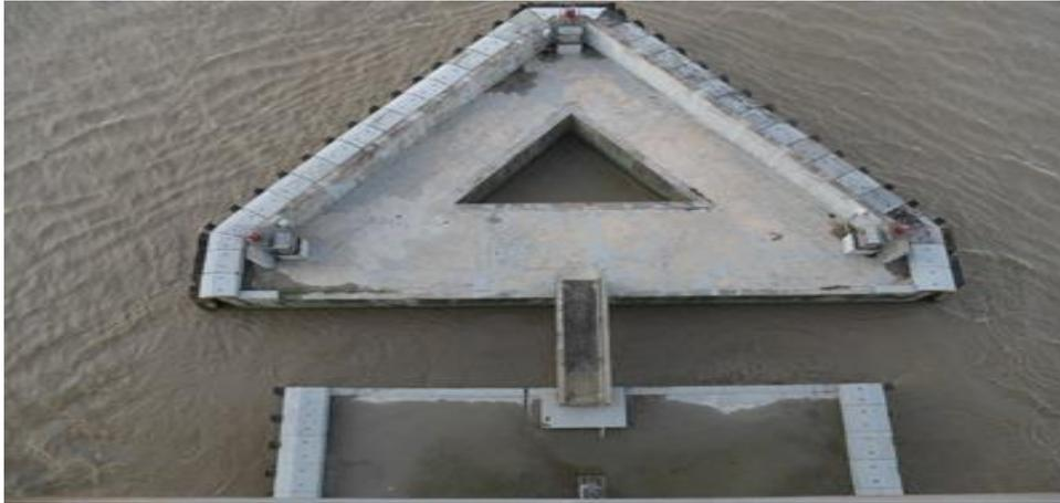
Figure 2: Basement of Bridge pier
