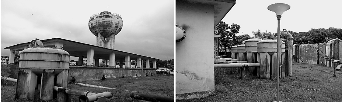
Figure 1: Gopalganj Water Treatment Plant
