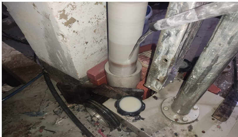
Figure 1: Core cutting process
