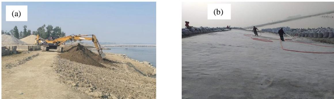
Figure 5: (a) Sloping procedure and (b) Geo-filter cloth for dumping of geo-bag
