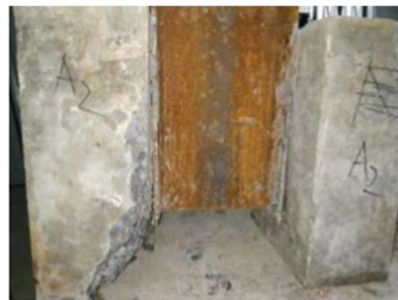
Figure. 5(b) Crushing of Concrete
