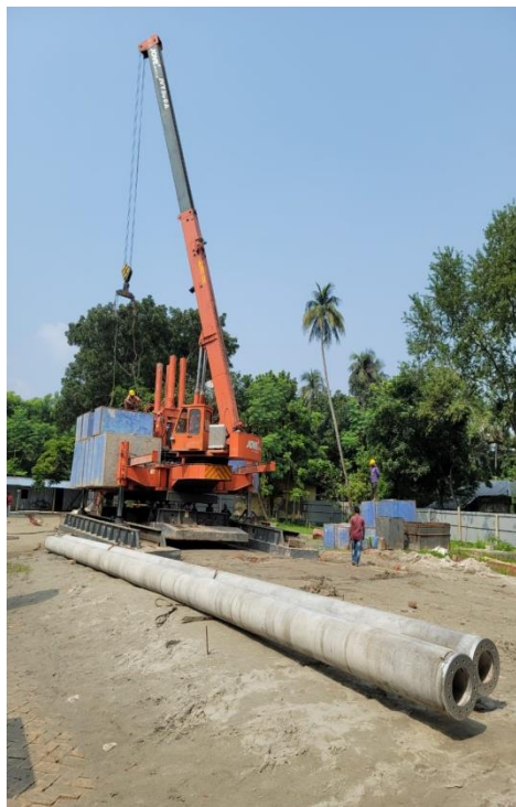
Figure 4: Hydraulic pile pressing machine
