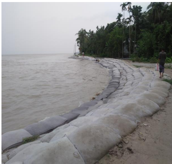
Figure 2: Primary stage of Geo Bag Filling Mulfatganj, Shariatpur district (10 March 2000)
