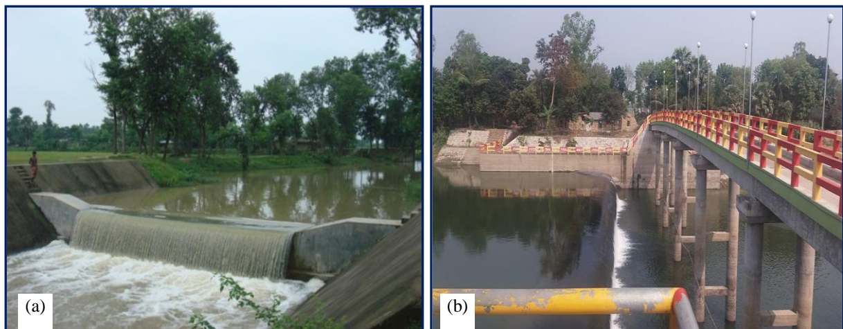
Figure 8: The re-excavated (a) Sarmaongla Khari with a cross dam under Godagari upazila and (b) a rubber dam at the Barnoi river under Puthia upazila of Rajshahi district
