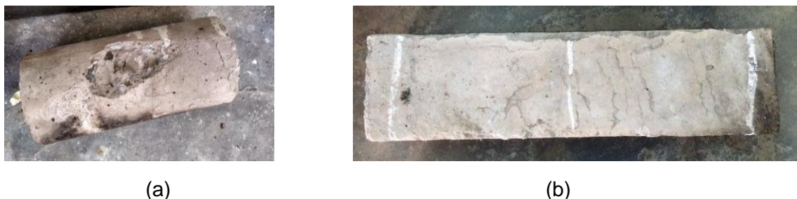
Figure 4: Spalling and cracks in specimens; (a) spalling in cylindrical specimen, (b) cracks in beam specimen.
