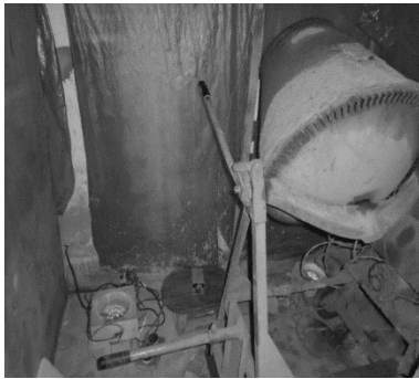
Figure 1: Mixing of Concrete
