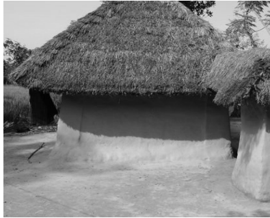
Figure 4: Existing housing condition in study area (Mud house)
